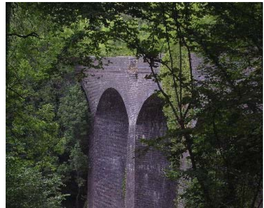
Midford Viaduct - will Nicolas Cage allow access via his path?
