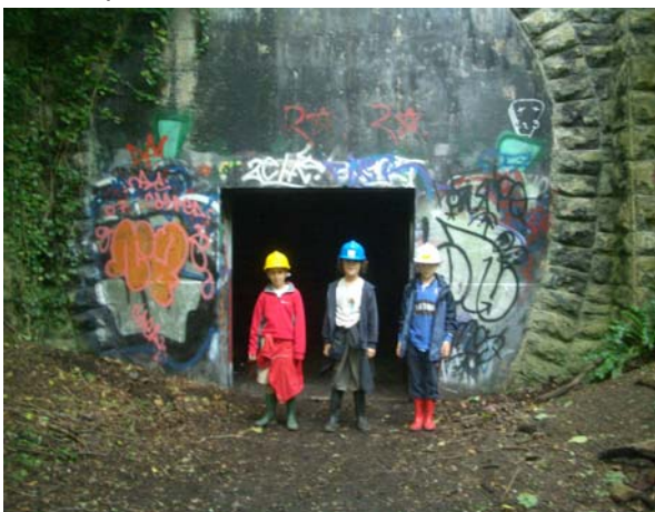
North entrance to Combe Down Tunnel
