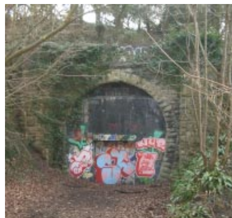
Devonshire Tunnel entrance
