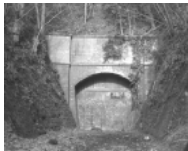
Cycling/walking through this tunnel?
